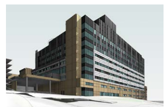
**Gosford Hospital Redevelopment, Sydney, Australia Size: 40,000 m 2 Year: 2013 - 2015
